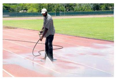
A large-size push broom with soft bristles or a power blower may be used to remove leaves and other debris and wet/dry vacuums, jet spray cleaners and power washers also may be used to clean and remove stains.
