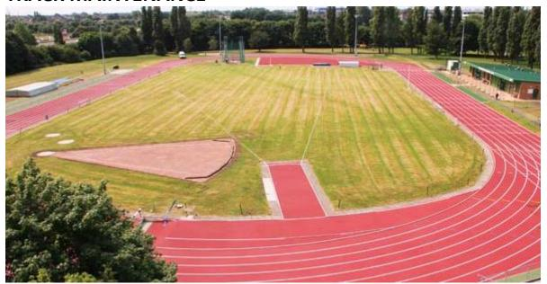
A well-designed, well-constructed and well-maintained track will provide a safe, resilient surface that will offer years of service. Note: a well-managed track will typically require a respray/re-top after 10years and 17years and a full surface replacement after 25years
